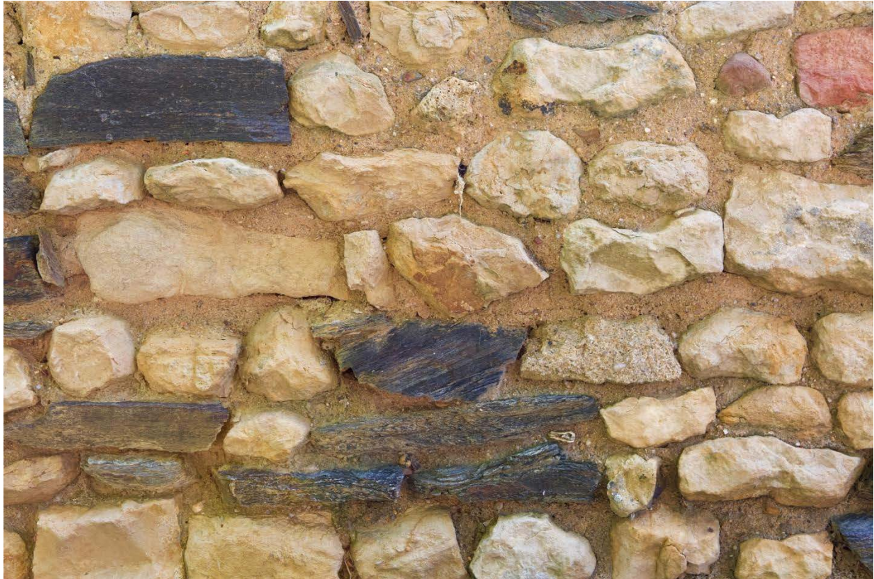
The walls tell the truth about the rocks in the ground: limestone, slate/schist, sandstone, silex—in one spot ...
